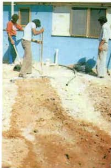
62. KOONIBBA, SA, AUSTRALIA Aboriginal gardeners dig an absorption trench from a kitchen sink outlet, in brick-hard ground. Trench is plastic-lined, manured, refilled, and planted. (See Number 63).
