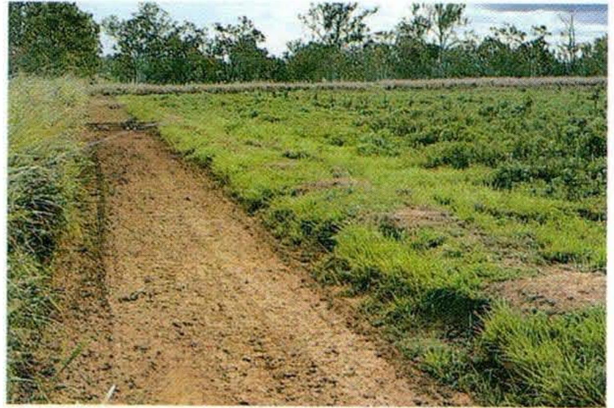
44. As for Number 43, here Bob has fitted a head drain with cross-stops to allow water to back up and flood the field to the right; again simple pipes are used, carefully levelled.
